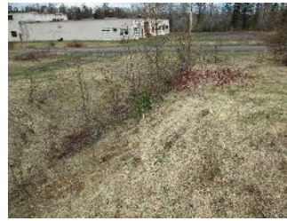
Ditch that receives parking lot drainage
