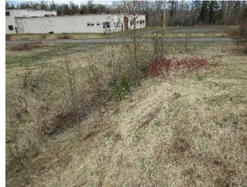
Ditch that receives parking lot drainage
