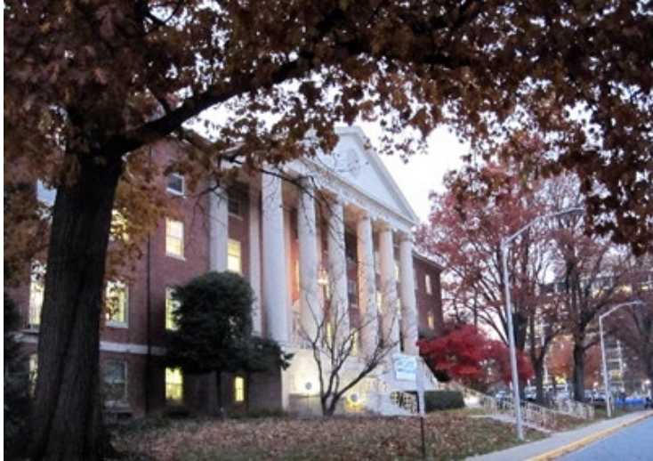
Figure 1. The James H. Shannon Building (Building One) on the NIH Campus in Bethesda, Maryland. Credit: NIH
